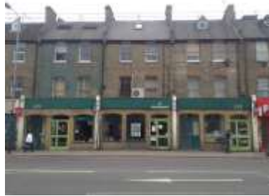
Photo 20: Intact Victorian fabric
